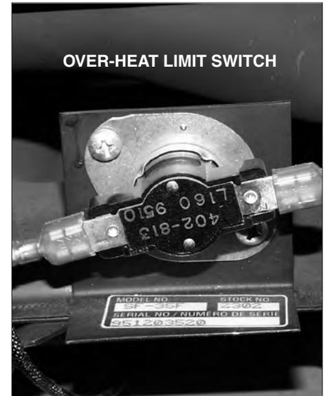
about six seconds after a delay of about 20 seconds from when the fan starts. If the ignition cycle does not start then it may mean that either the sail switch or limit switch, or both, are defective. If they are not then the ignition control board may be defective and will need replacing.
