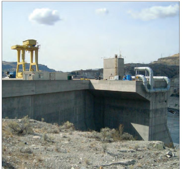
Dam is a gravity dam and has a length 5,223 feet. Its height is 550 feet. It required 11,975,521 cubic yards of concrete. It generates 6,809 megawatts.
